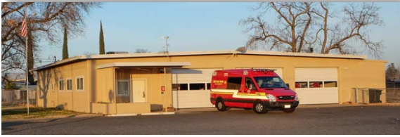
STATION #112 6801 34th Street North Highlands
