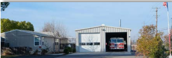
STATION #117 7961 Cherry Brook Drive Elverta
