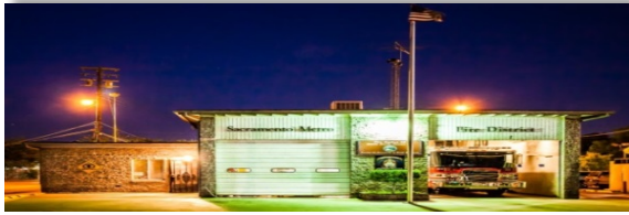
STATION #42 5608 North Haven North Highlands
