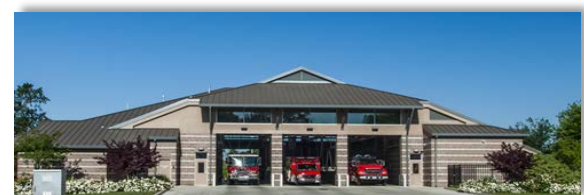
STATION #111 6609 Rio Linda Blvd. Rio Linda
