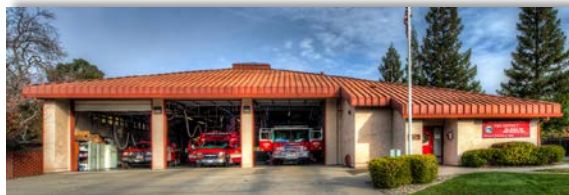
STATION #105 2691 Northrop Avenue Sacramento
