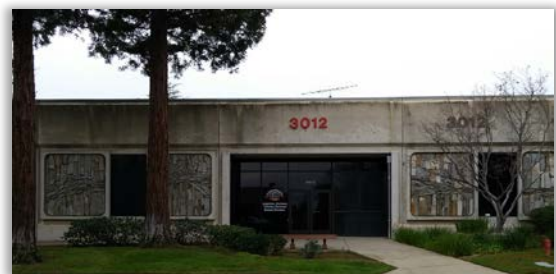
LOGISTICS/TRAINING/SAFETY 3012 Gold Canal Drive Rancho Cordova
