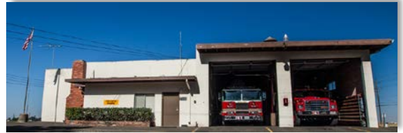
STATION #116 7995 Elwyn Avenue Elverta
