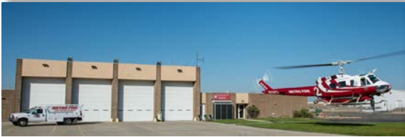
STATION #115 4727 Kilzer Avenue McClellan
