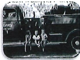
Elverta Fire District
