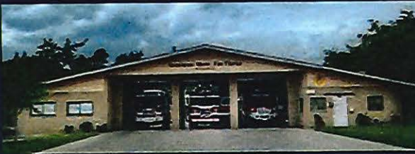
STATION 23 REPLACEMENT Citrus Heights
