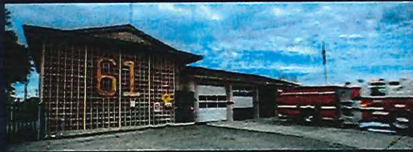
STATION 61 REPLACEMENT Rancho Cordova
