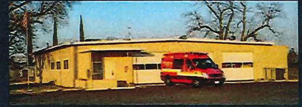
STATION 112 REPLACEMENT North Highlands
