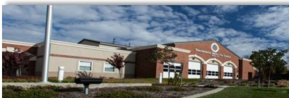
STATION #29 8681 Greenback Lane Orangevale
