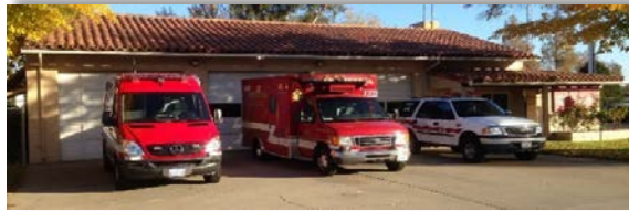
STATION #102 4501 Marconi Avenue Sacramento
