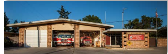
STATION #103 3824 Watt Avenue Sacramento
