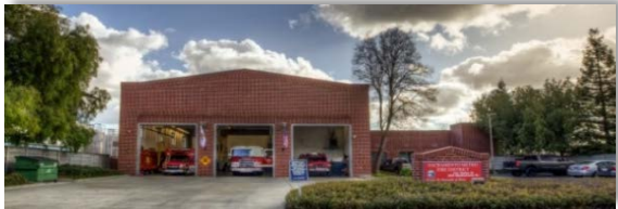
STATION #51 8210 Meadowhaven Drive Sacramento
