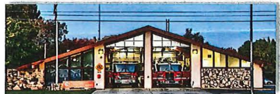
STATION #62 3646 Bradshaw Road Sacramento
