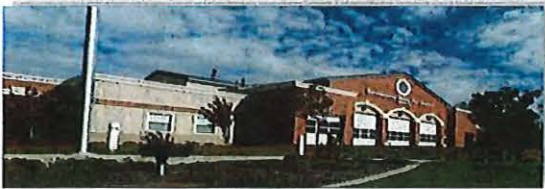
STATION #29 8681 Greenback Lane Orangevale
