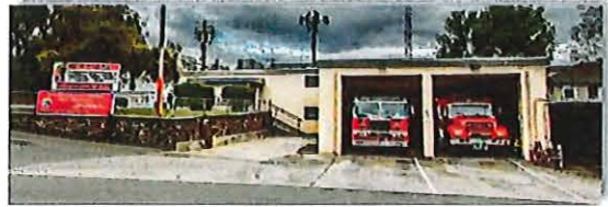
STATION #31 7950 California Avenue Fair Oaks
