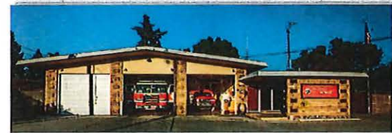
STATION #103 3824 Watt Avenue Sacramento
