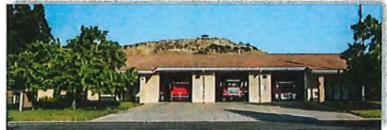
STATION #59 7210 Murieta Drive Rancho Murieta
