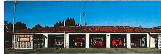
STATION #101 3000 Fulton Avenue Sacramento
