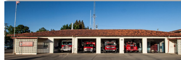
STATION #101 3000 Fulton Avenue Sacramento
