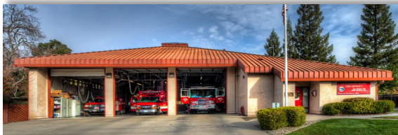
STATION #105 2691 Northrop Avenue Sacramento
