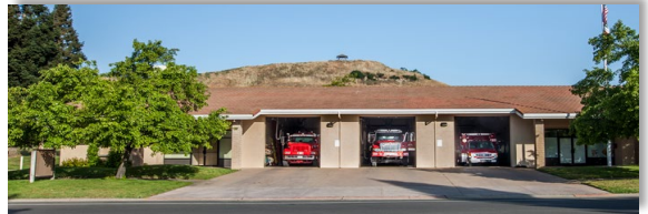
STATION #59 7210 Murieta Drive Rancho Murieta
