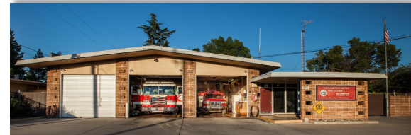
STATION #103 3824 Watt Avenue Sacramento
