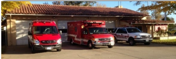
STATION #102 4501 Marconi Avenue Sacramento
