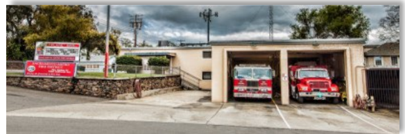
STATION #31 7950 California Avenue Fair Oaks
